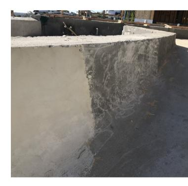
**MiraFlex Membrane C Flexible Cementitious Waterproofing** creates a seamless waterproofing vessel that reduces reflective cracking and does not age harden. The vapor permeable membrane is ideal for interior or exterior exposure.
