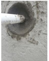
**MiraPatch WP** is a hydraulic water plug for active leaks, packing pipe penetrations, and other applications requiring fast setting and rapid strength gain in full immersion service conditions.
