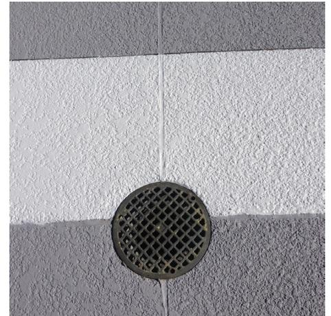
Other Miracote products were used to repair or level concrete and color and seal the deck, such as MiraPatch RM 1 and MiraGard HD 100.
