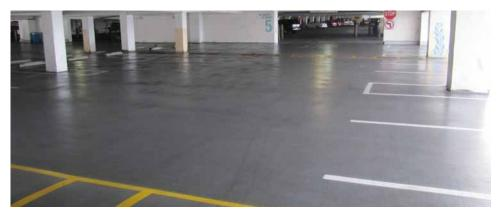
Hard Powder contains aluminum oxide aggregate for enhanced abrasion resistance on turn lanes and entrance and exit ramps.
