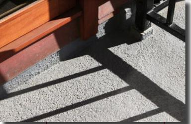
resistance, making it ideal for outdoor applications. Next, a splatter coat of Miracote MPC was applied with a hopper gun. After allowing this coat to cure to a heavy, semi-dry orange peel texture, a knockdown finish was achieved by taking a flat trowel and skimming off, literally "knocking down", the high spots of the coating.
