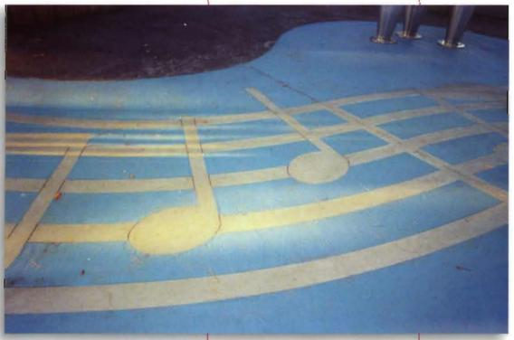
suggested surfacing the existing concrete with Miracote MPC, a polymerized cementitious material designed specifically for heavy pedestrian and vehicular traffic. He then recommended Miracote Colorbond as the topcoat. Colorbond is a single component acrylic finishing topcoat with excellent durability and resistance to adverse weathering conditions.
