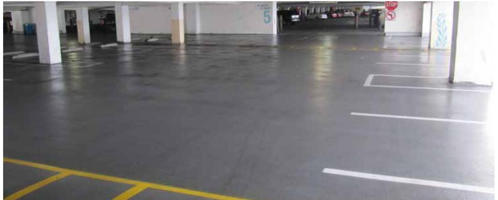
Hard Powder contains aluminum oxide aggregate for enhanced abrasion resistance on turn lanes and entrance and exit ramps.
